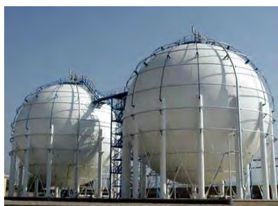
High Pressure LPG Tank with ambient Temperature
